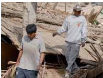
The Development Office - Procura de la Compañía de Jesús distributed 190 tonnes of food and other supplies. Attending to 60 emergency canteens and 3,500 families in the fourteen sectors organised by the Parroquia Cristo Rey, in the Pueblo Nuevo district of Chincha.
